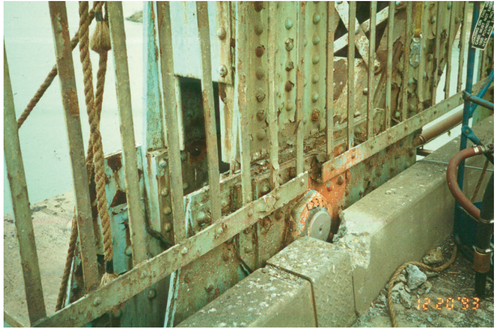
Figure 8.6.60 Suspended Span Pin
