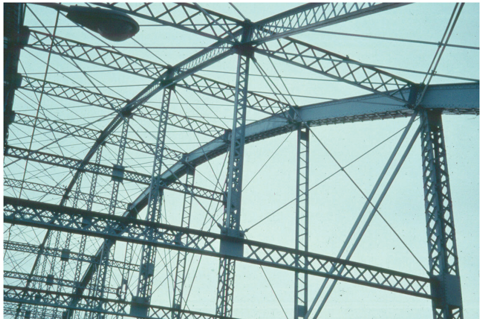
Figure 8.6.39 Sway Bracing
