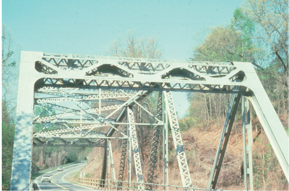
Figure 8.6.40 Portal Bracing
