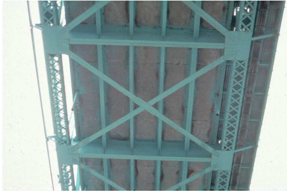
Figure 8.6.36 Lower Lateral Bracing
