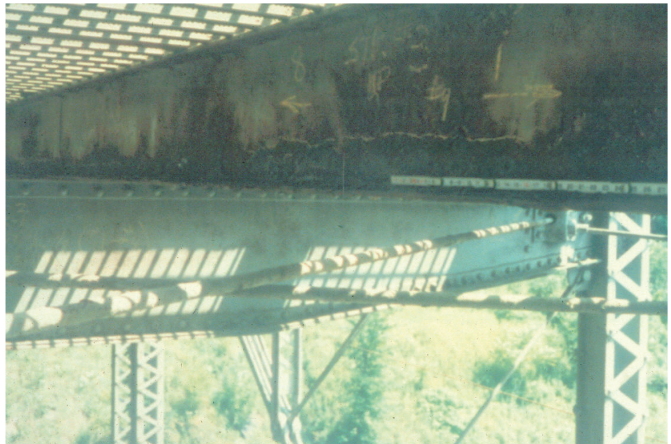
Figure 8.6.54 Corroded Stringer
