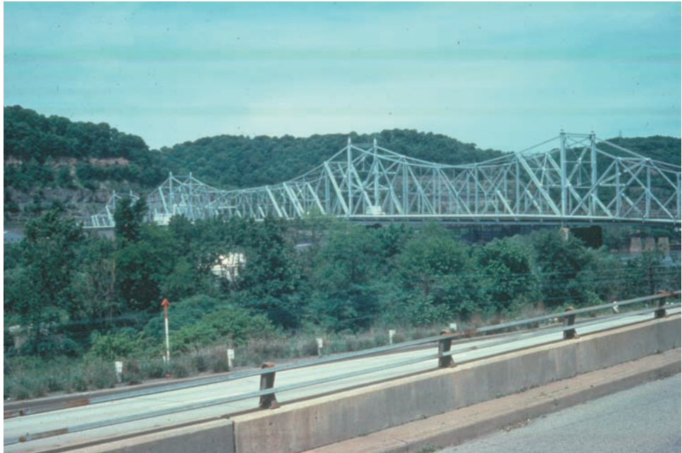
Figure 8.6.15 Cantilever Through Truss
