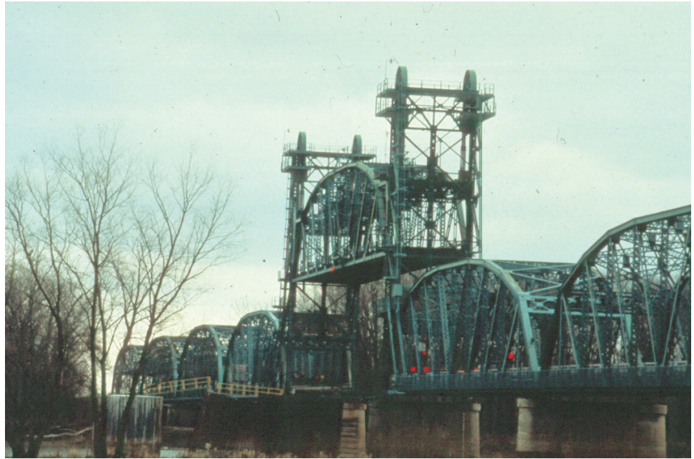
Figure 8.6.8 Vertical Lift Bridge
