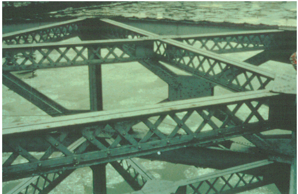
Figure 8.6.35 Upper Lateral Bracing
