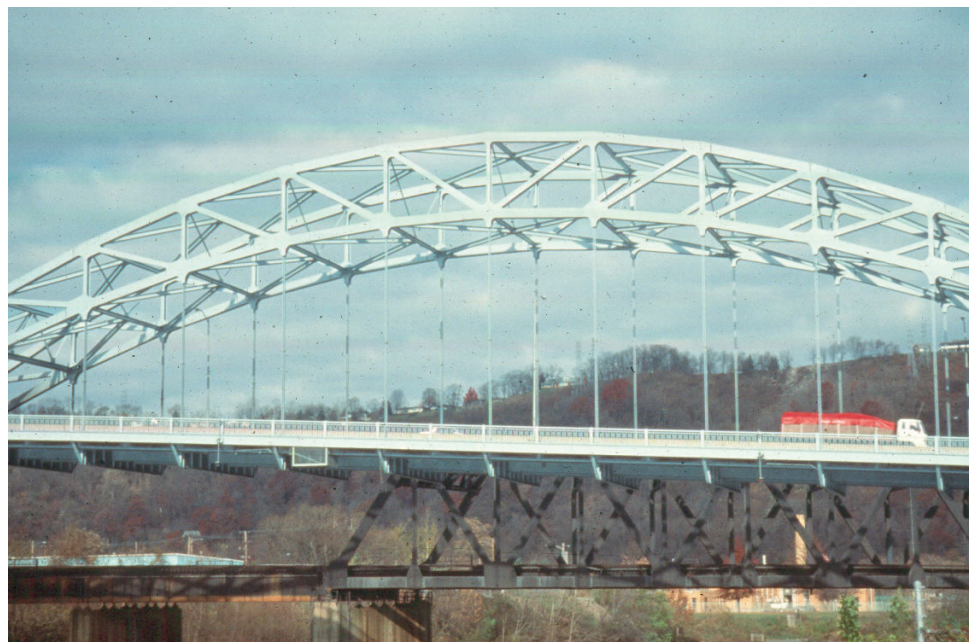
Figure 8.6.7 Arch Bridge with Stiffening Truss
