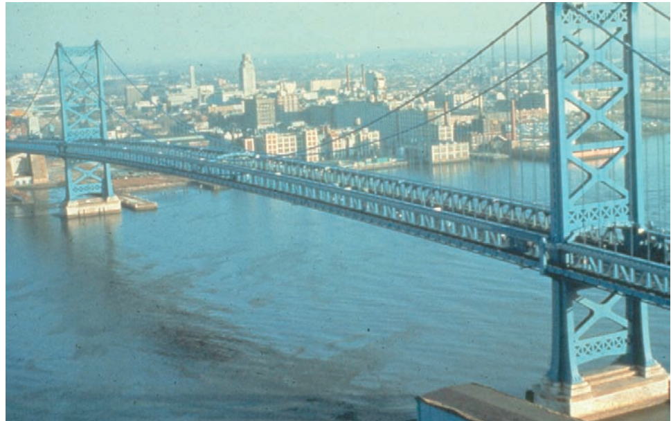
Figure 8.6.6 Suspension Bridge with Stiffening Truss
