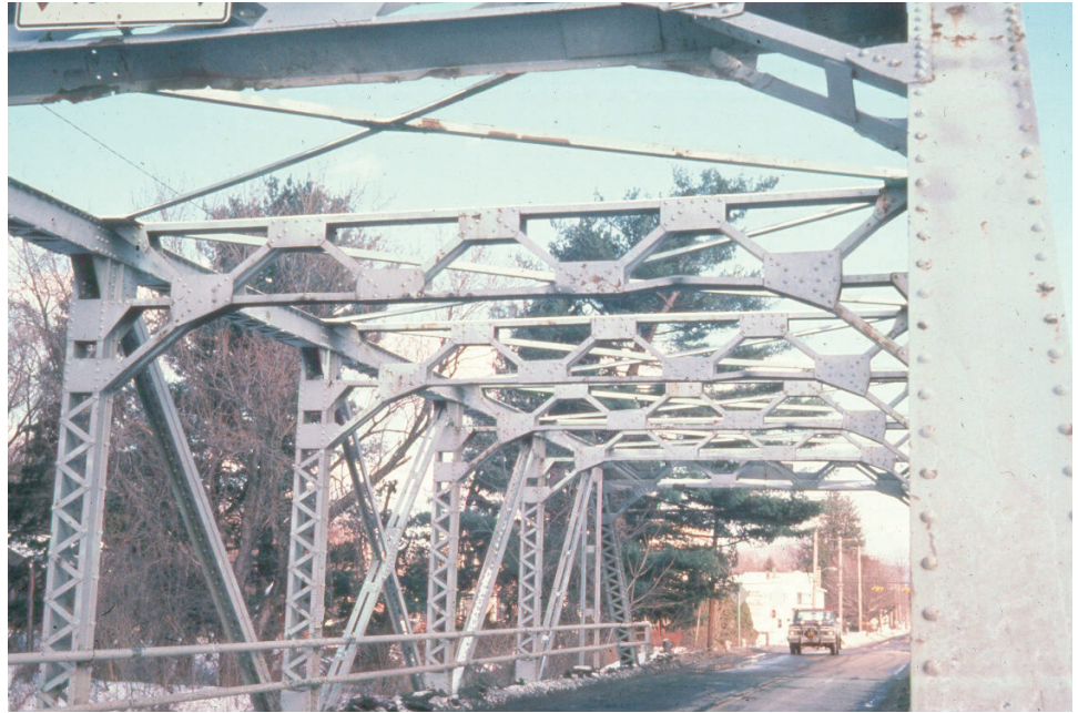
Figure 8.6.38 Sway Bracing
