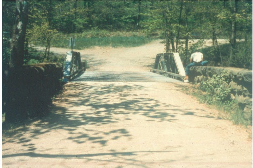
Figure 8.6.4 Pony Truss
