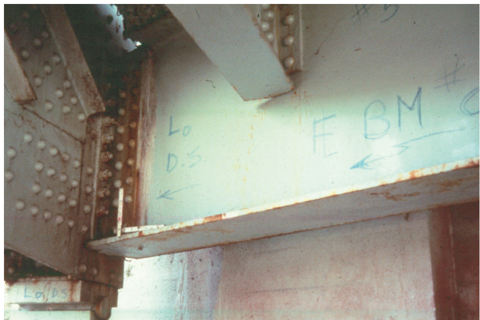
Figure 8.6.59 Clip Angles at Floorbeam and Stringer Connections
