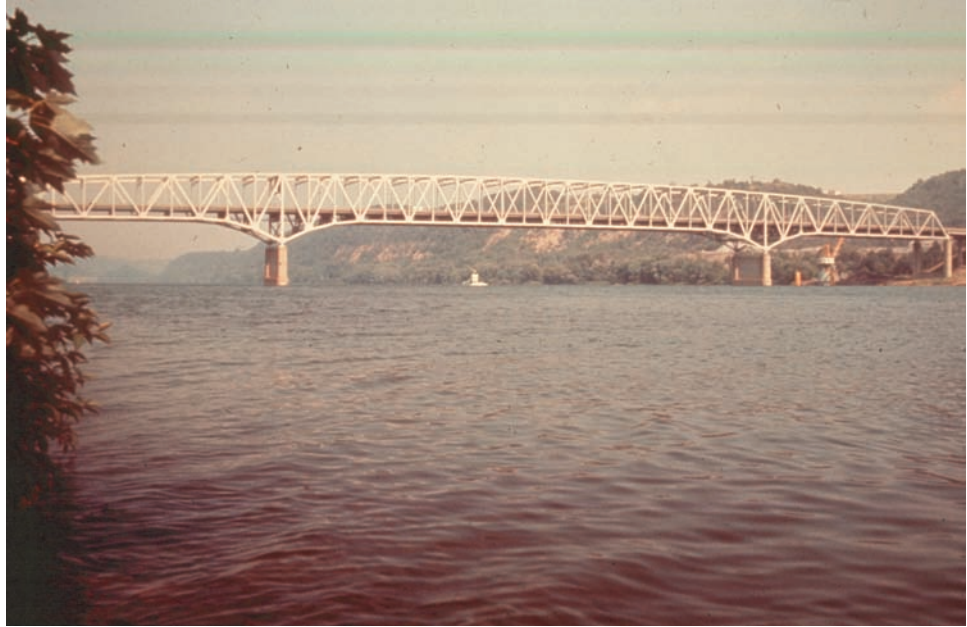
Figure 8.6.14 Continuous Through Truss
